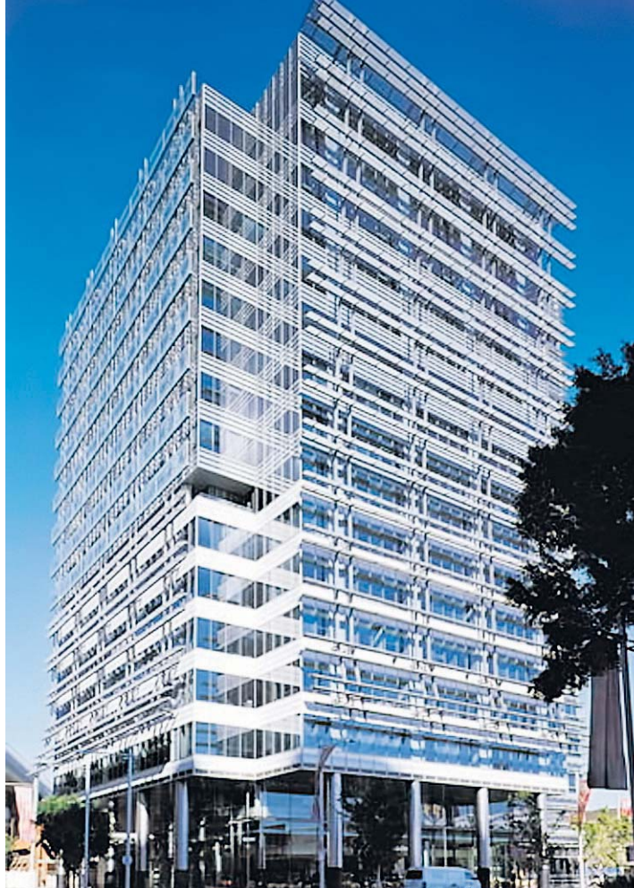
Shining asset: The head office of KPMG at 10 Shelley Street, Sydney, is among five office buildings GPT Group will buy.
